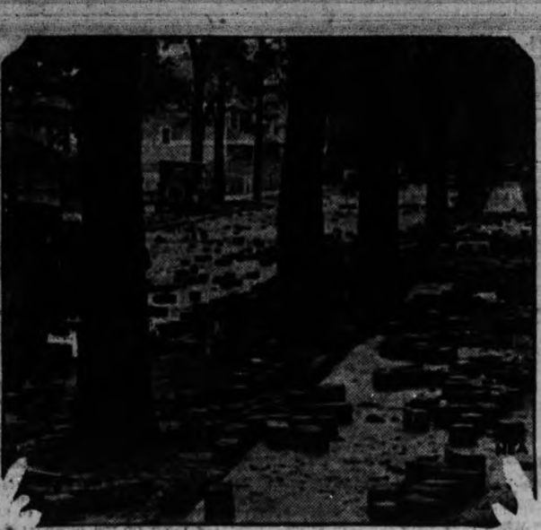
WHAT VICTORIA BLOCK-PAVED STREETS MAY LOOK LIKE SOON—They had a heavy rain in Detroit—almost a cloud-burst—and it flooded dozens of streets. Streets that were paved with wood or composition blocks suffered heavily, as the blocks floated away and were scattered all over the city when the waters subsided.
